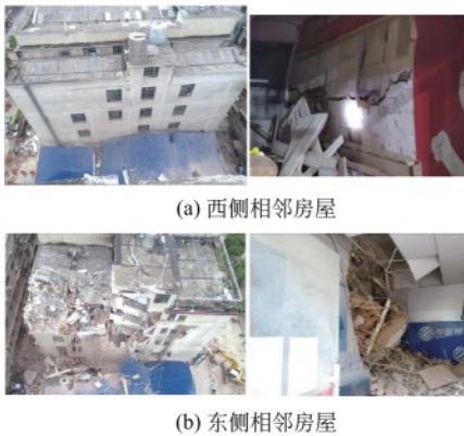
图5 两侧相邻房屋整体及一层墙受损情况 Fig. 5 Overall and first floor wall damage to adjacent houses on both sides
