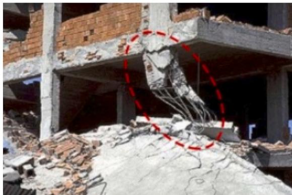
Fig. 1. Example of collapse caused by column impact failure [41].
