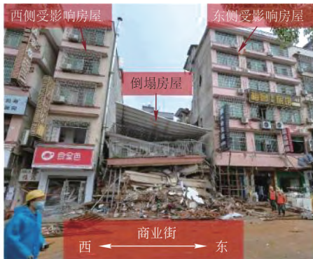
图4 房屋倒塌后状态 Fig. 4 State of the structure after collapse
