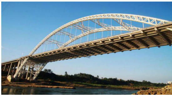
Fig. 1 Photograph of the Laihua Bridge
