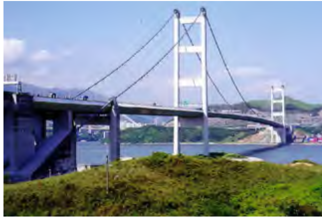
Figure 2. Tsing Ma Bridge.
