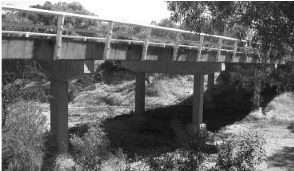
Fig. 2. View of MRWA bridge no. 3014
