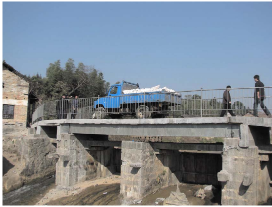
Fig. 9. Truck loading test of Leiyang Bridge
