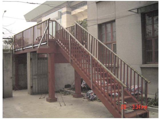
Fig. 5. Modern bamboo pedestrian bridge
