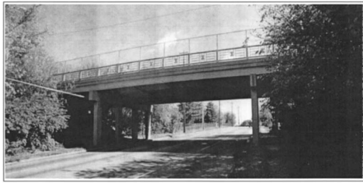
Fig. 1. Seymour Bridge, Cincinnati, Ohio
